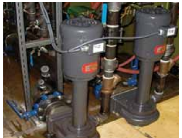
“Zero tank” return pump
